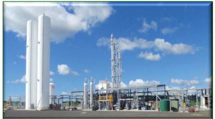
A natural gas liquefaction plant, similar to one proposed.
